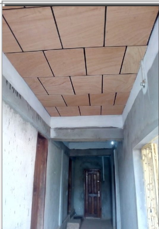
Ceiling in Hallway
