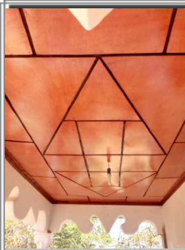
Veranda: plastering, varnished ceiling & painted window-hoods to protect wooden window against rain
