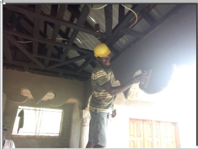
Veranda: plastering, varnished ceiling & painted window-hoods to protect wooden window against rain
