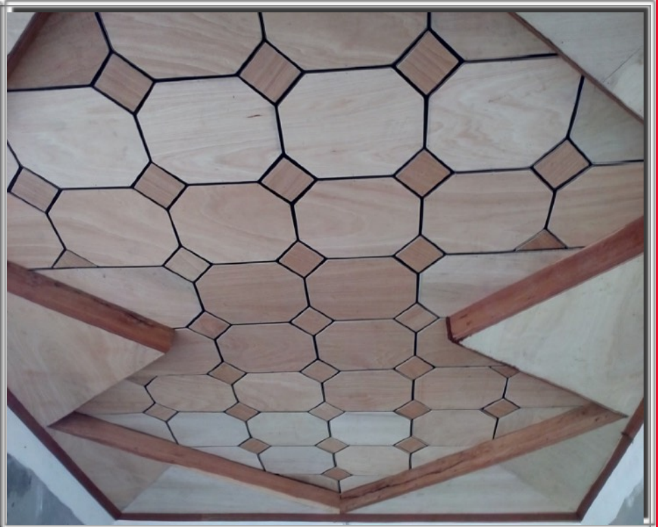
2 layer deep, mosaic ceiling design
